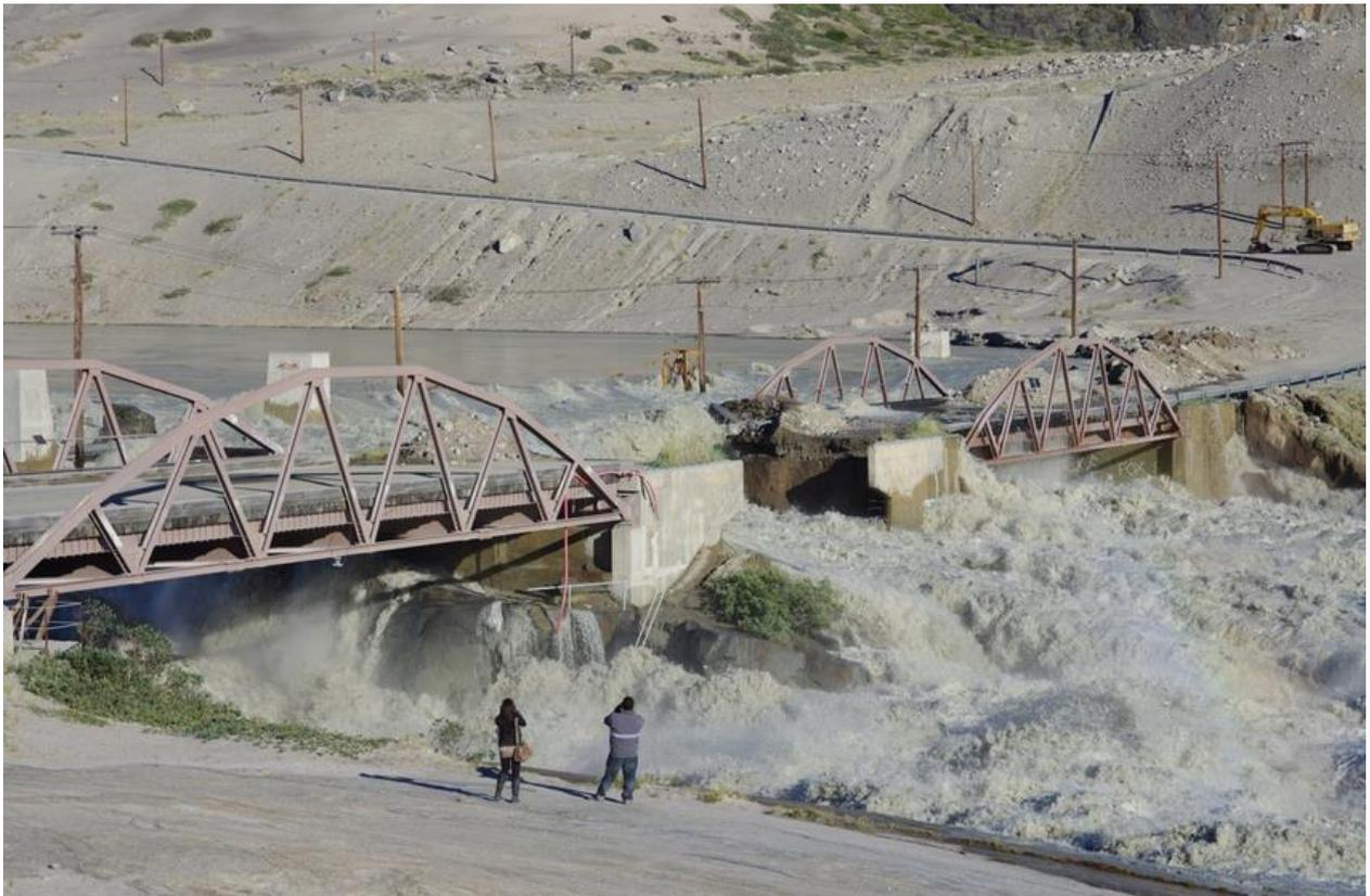
Figure 4: The washout of the Watson River Bridge in Kangerlussuaq, Greenland following a record-setting proglacial discharge (Mikkelsen *et al*. 2016).
